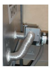
Typical ClevaFlex Air Handling Duct application:
